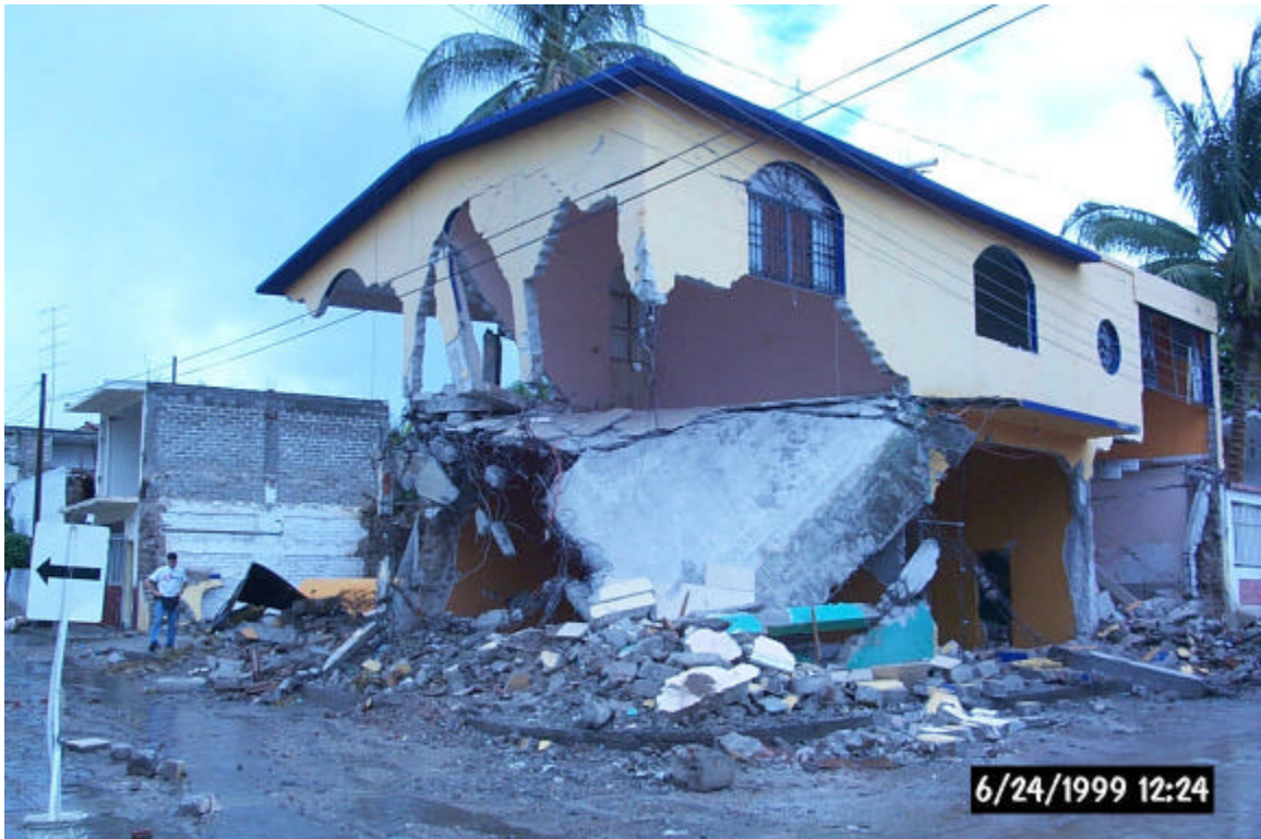
Figure 4.10 Damaged modern reinforced concrete structure in Acatlán de Osorio.
